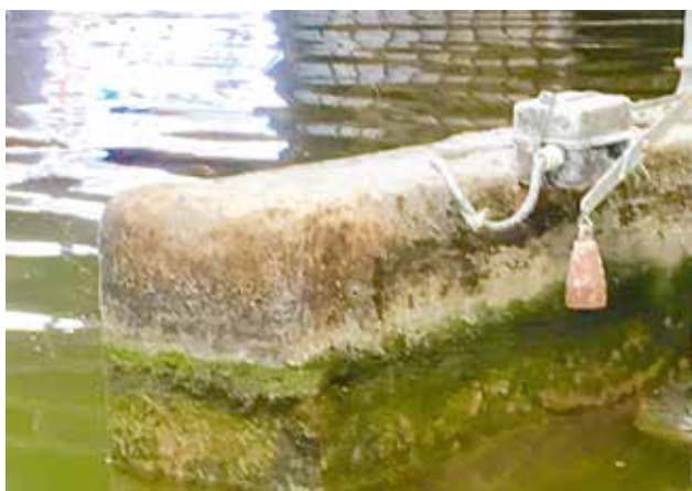
Figure 5: Wall of treated water storage chest showing growth of algae.
