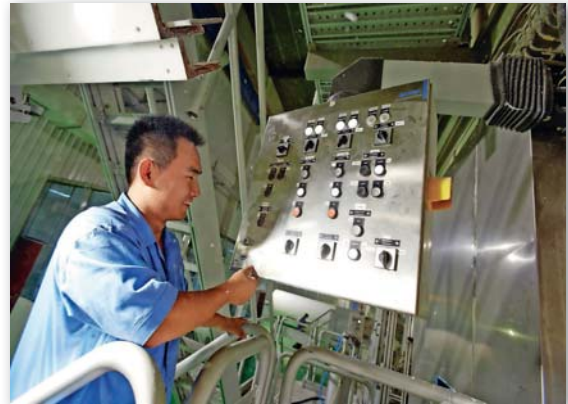
ANDRITZ automation installed at Sun Paper Yanzhou (two 2000 m/min tissue machines).
